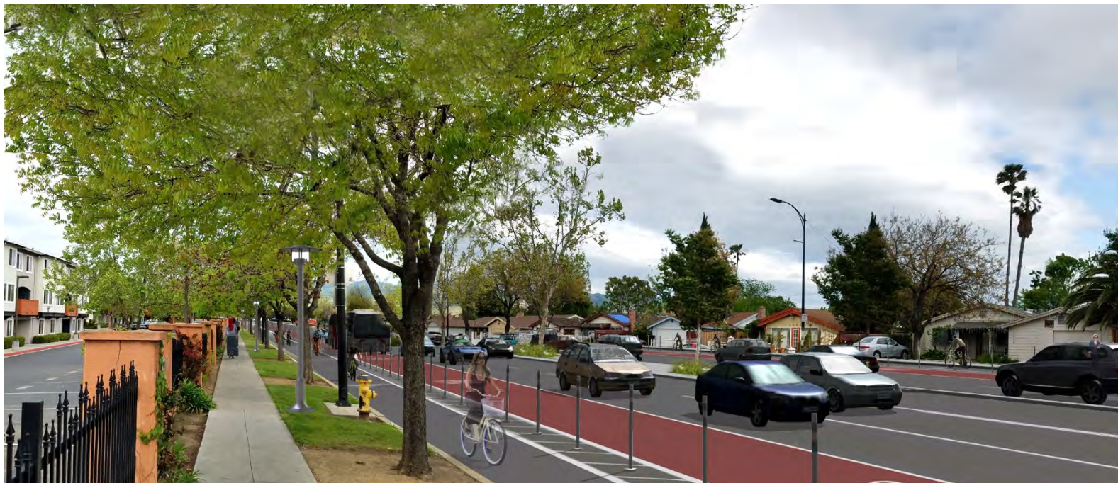
Story Road – This is a typical rendering of the segment improvements on Story Road, which converts the outside travel lane to a bus only lane and accommodates a separated bikeways. The separated bikeways is shown here with a striped buffer and flexible posts.
