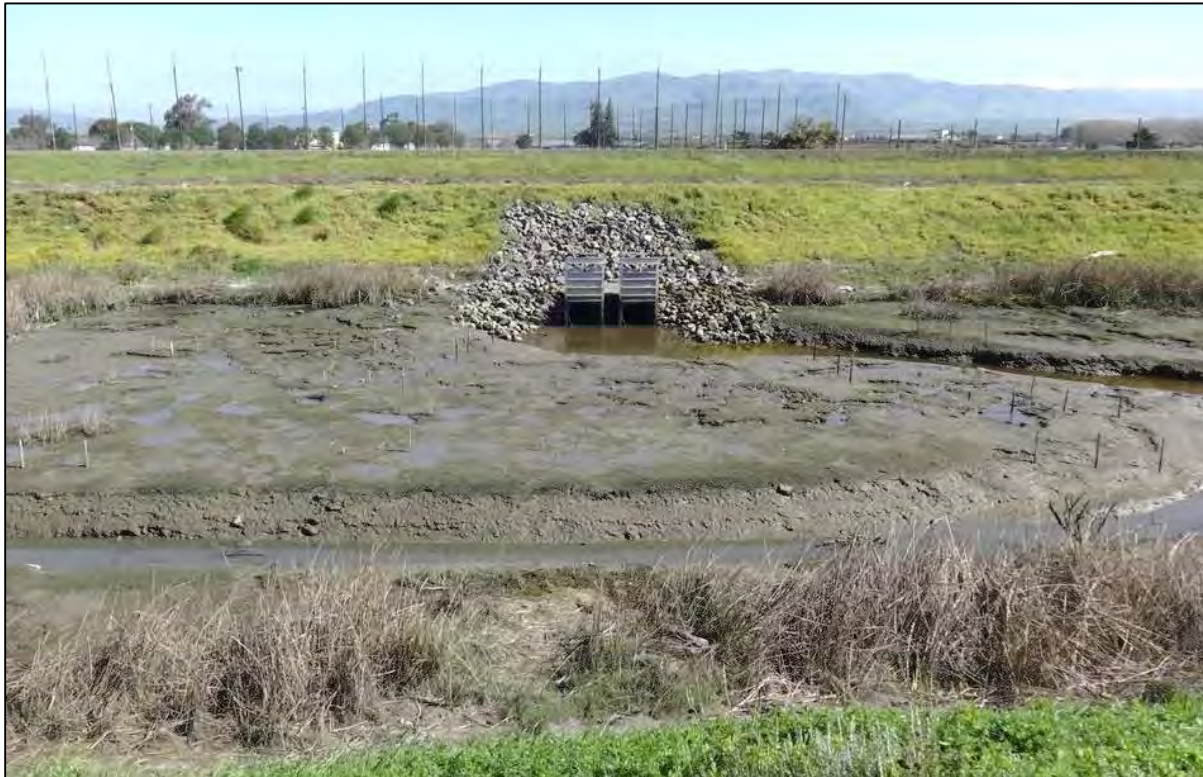
Figure 6. Tasman Site during Low Tide (Photo of Northern Culverts on 12 March 2015)
