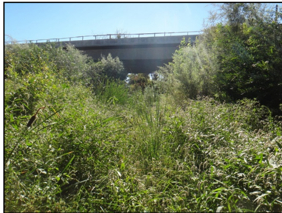
Photo 4. View of In-Channel Wetland 2, looking southwest from the New Roadway Bridge Crossing
