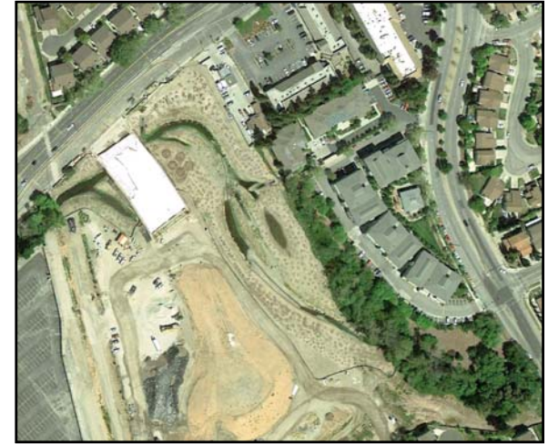
C. April 2013, 6 months after channel construction.
