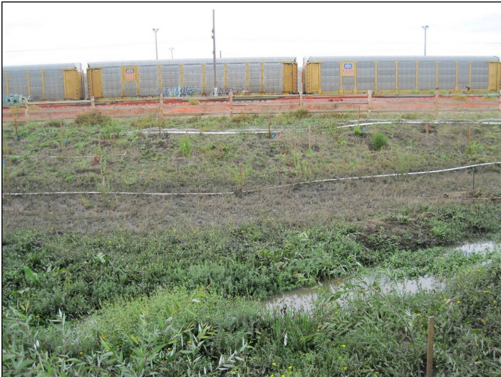
Figure A-8. Photopoint 23, looking across the channel from the west bank to the east bank (October 2011).
