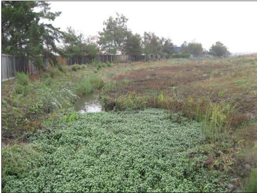
Photo 1. Photo-point 1, looking upstream from the culvert at the downstream project extent (October 2011)
