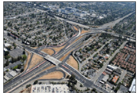
I-280/I-880/Stevens Creek Blvd Improvement Project completed August 2015.
