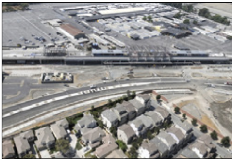
Berryessa BART Station getting final touches of plaza and roadway.
