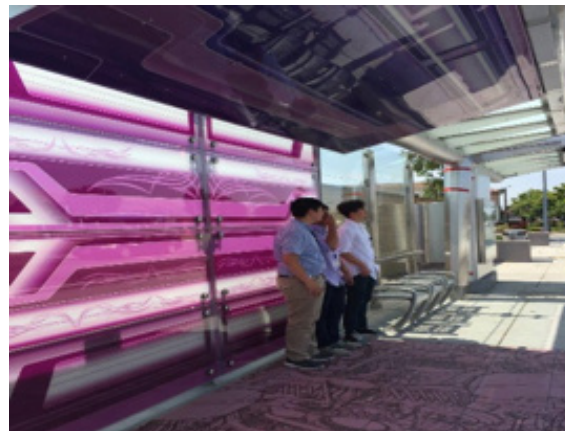
Story Road Eastbound BRT Station inspired by lowrider car culture in east San Jose.
