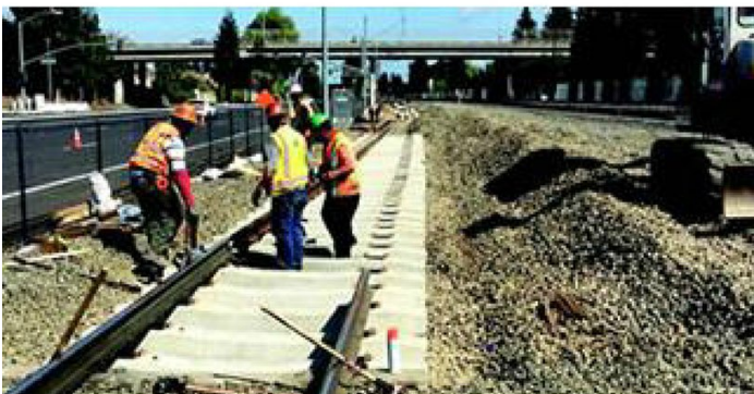
Award Winning Mountain View Double Track Project
