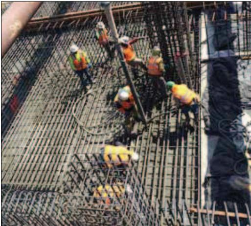
VTA's BART Silicon Valley Extension - Crews pouring concrete for the Milpitas Station foundation slab.
