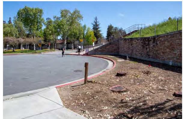
Sidewalk gap at end of River Oaks Place, which connects to Guadalupe River Trail
