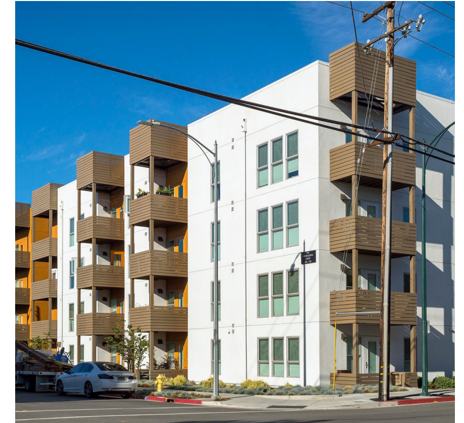
Foundry Commons, San José
