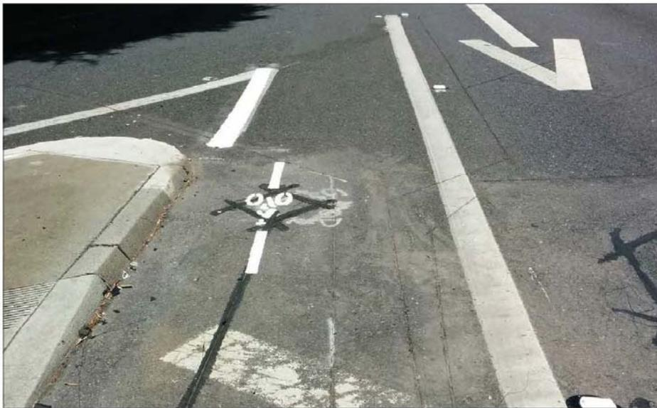
b. View of a bike detector embedded in a bike slot. The purpose of a bike detector is to detect a bicyclist approaching an intersection and communicate with the traffic signal cabinet to provide enough time for cyclists to safely cross an intersection.
