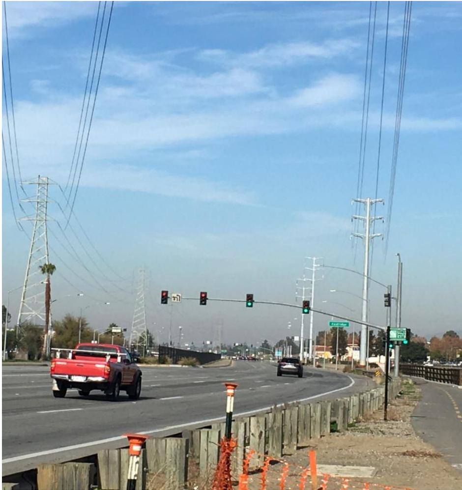
Image shows the PG&E transmissions line on the left being relocated and replaced by new design and new line on the right.
