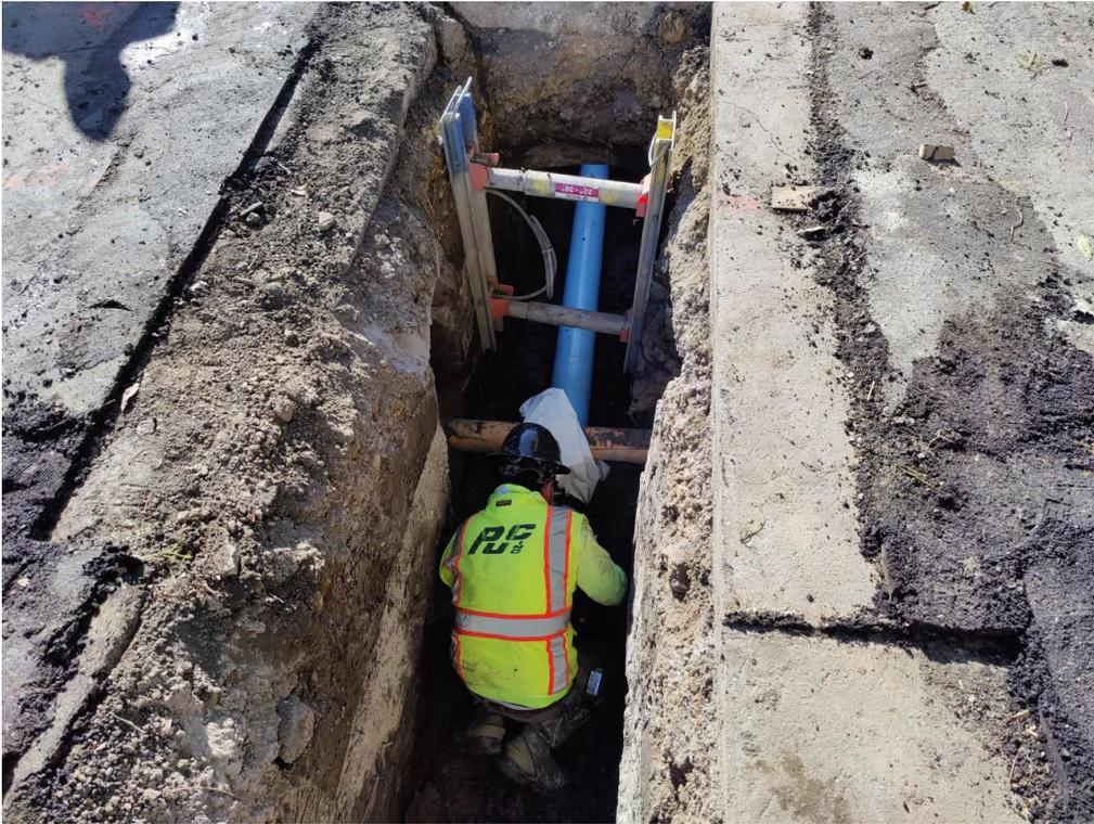
Image on the right of crews relocating a water line near Highwood and Capitol Avenue.
