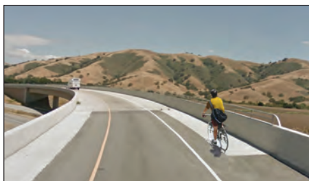
Eastbound SR 152 flyover of SR 156 has wide right-hand shoulder with bicycle railing to accommodate the bicyclists on this route.
