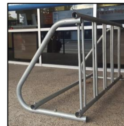
Wheel bender-type racks should be replaced
