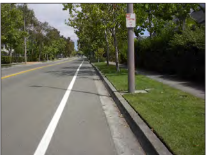
Bike lane-parking prohibited.
