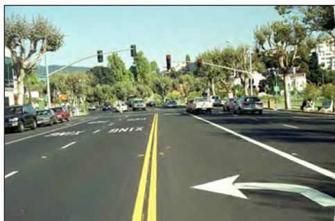
Typical left-turn pocket at a signalized intersection.
