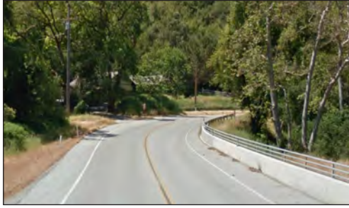
Uvas Creek Road with widened shoulders
