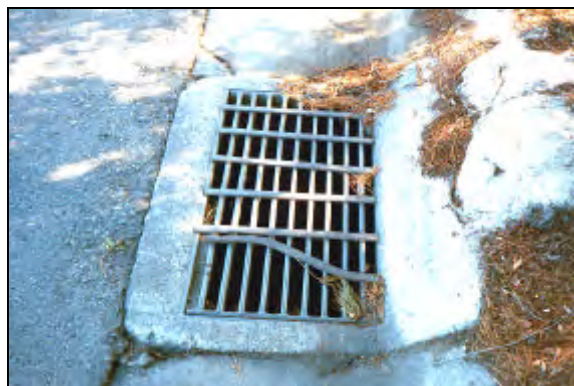
Retrofitted parallel bar grate, San Tomas Expwy
