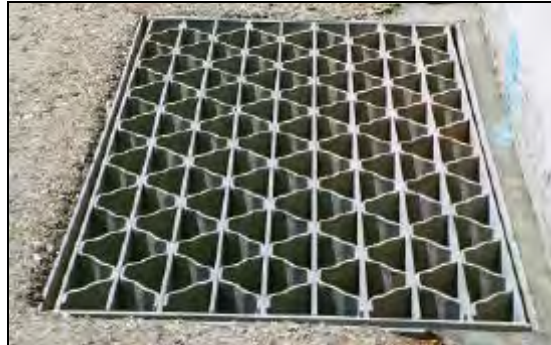
County Type 1C ("honeycomb") grate
