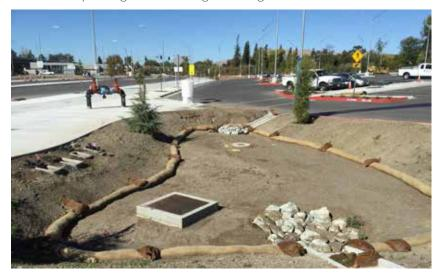
**Figure 6:** Bioretention basin is inadequately protected with only fiber rolls. Note the accumulated sediment filling the rock riprap and discoloring the soil media on the left half of the basin.
