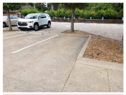
Figure 12: Pervious pavement in a parking lot.
