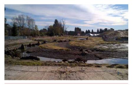
Figure 4: Final site erosion controls with jute blankets and hydroseed.
