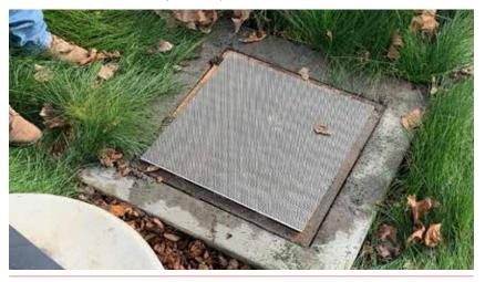
Figure 19: 5mm Trash Screen on Bioretention Basin
