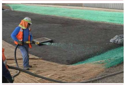
**Figure 7:** Bioretention basin is adequately protected from construction run-on using temporary hydromulch and erosion control blanket.
