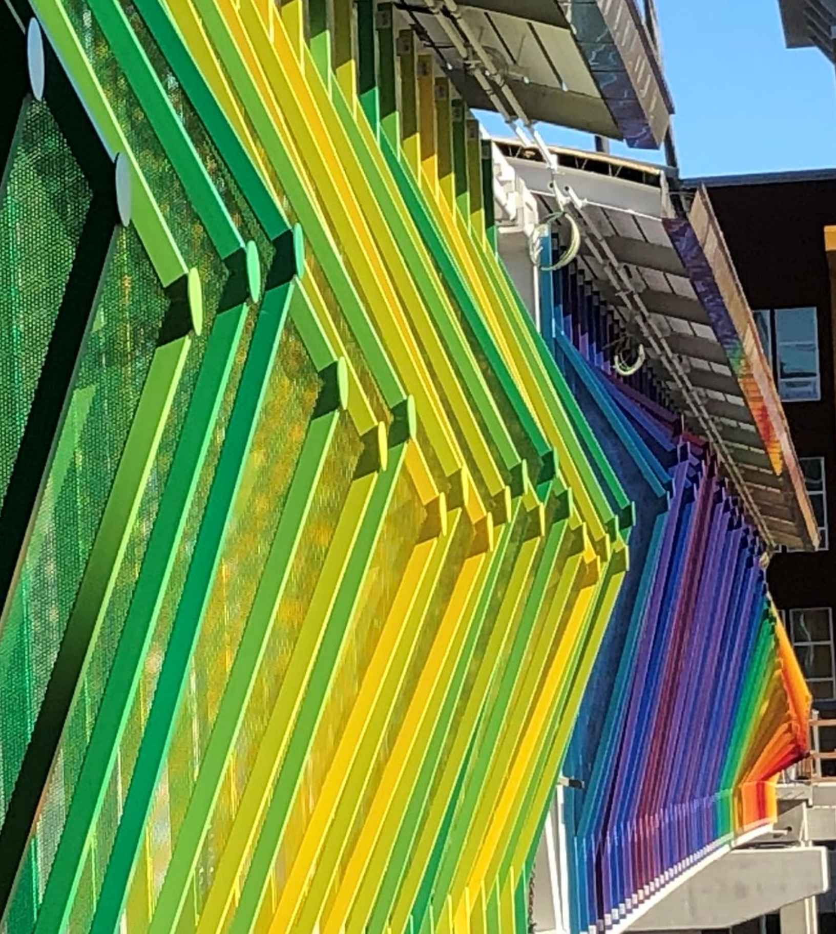
Pedestrian bridge at Milpitas Transit Center
