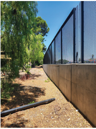
New retaining wall for the new separation bike & pedestrian pathway.
