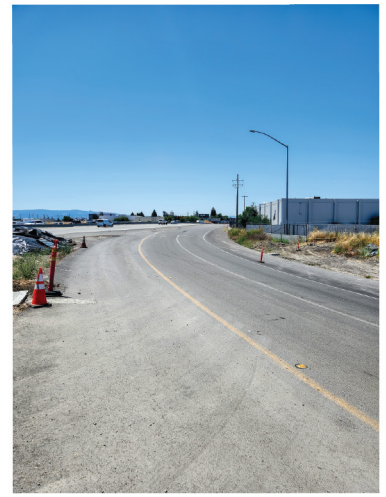
New Northbound on-ramp US 101 from De La Cruz Blvd.
