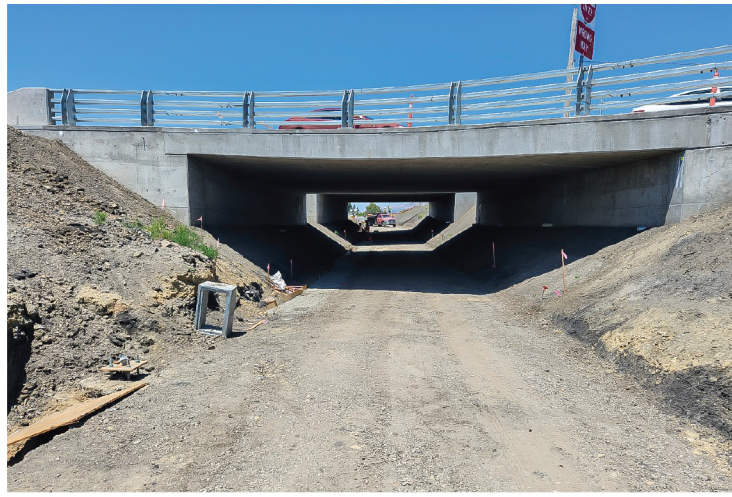
New Pedestrian undercrossing beneath the Southbound off & on campus.
