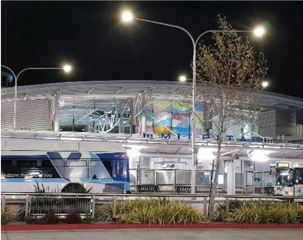
Milpitas BART Station
