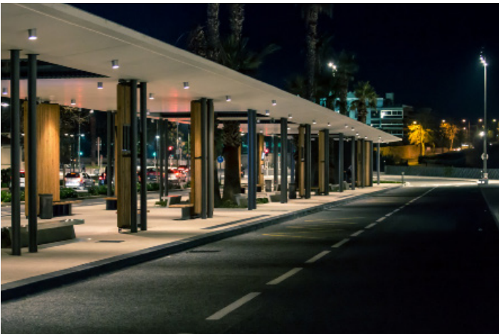
Adequate Lighting - Photo Credit: Franck Michel, Flickr
