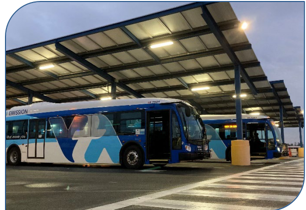
VTA Buses Under Solar Canopies
