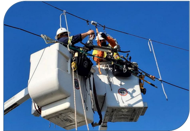
VTA Workers Repairing Overhead Lines
