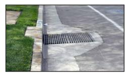
Grate wider than gutter pan reduces usable bike lane width to less than the 36 in. min. specified in HDM §301.2.
