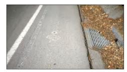
This drainage grate located off of the shoulder will not force cyclists into the travel lane in order to avoid it.
