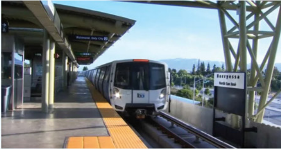
State of California awarded $375 million to the SCVTA for its BART extension into Downtown San Jose and Santa Clara.
