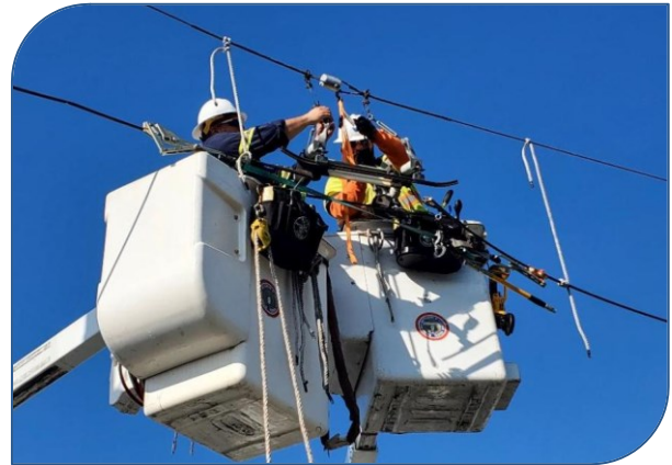
VTA Workers Repairing Overhead Lines
