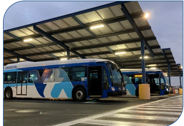
VTA Buses Under Solar Canopies
