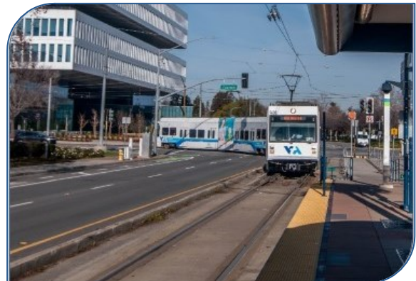
Tasman Grade Crossing
