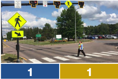
1 1 High Visibility Crosswalks
