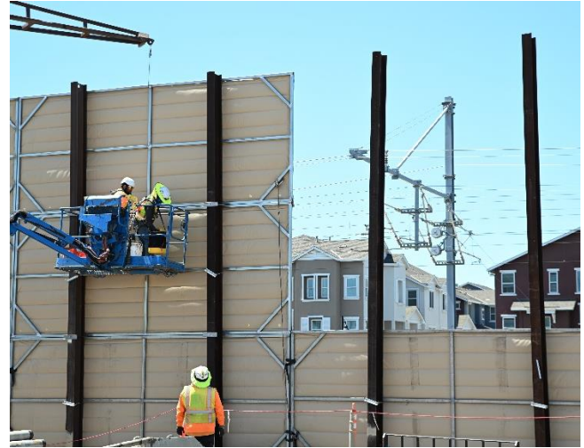
Noise curtain installation next to the train tracks to help reduce noise for nearby residents.
