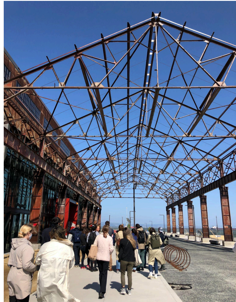
Figure 9. Example Structural frame creative reuse — Pier 70 building 15 over 22nd Street in San Francisco
