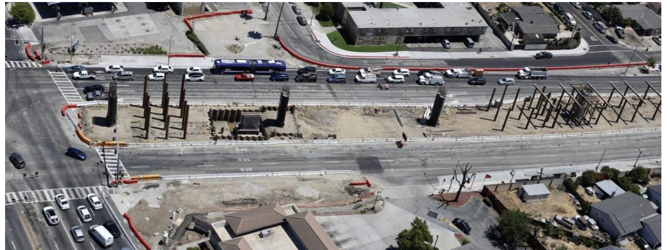
Bridge foundation work south of Story Road
