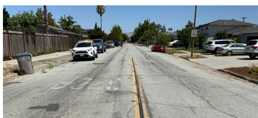
Chesbro Avenue, before - City of San Jose
