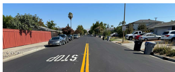
Chesbro Avenue, after - City of San Jose
