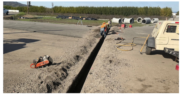
Underground drainage and utility improvements.
