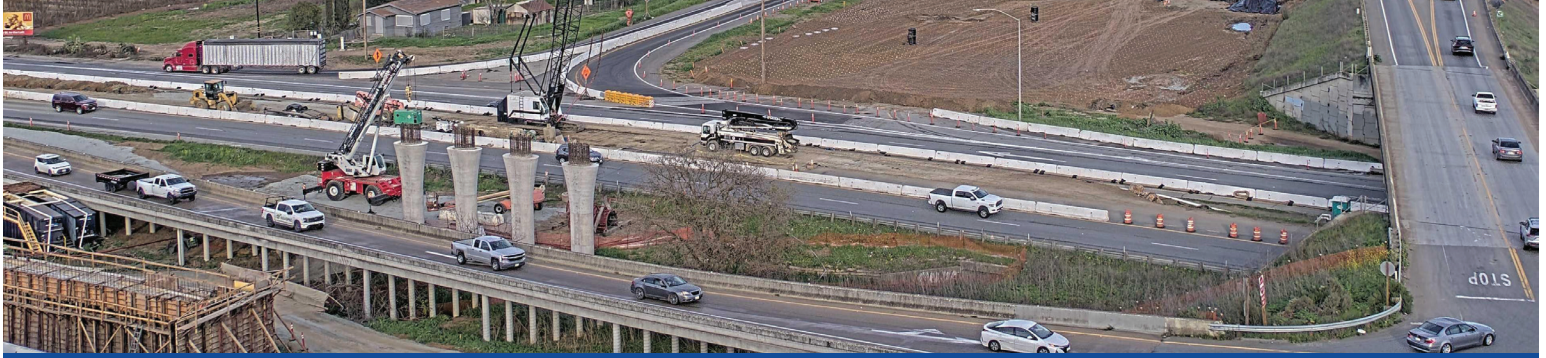
Figure 1: This photo shows the new US 101 overcrossing (separation structure) columns, and existing SB off-ramp bridge
