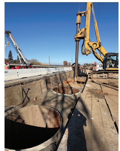
Deep foundation and bridge support work underway.
