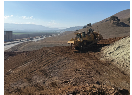
Early grading and site preparation near the interchange.
