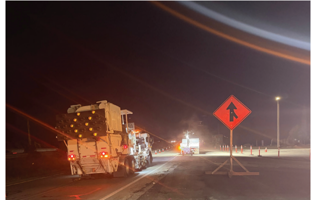
Night work and temporary traffic control near the interchange.
