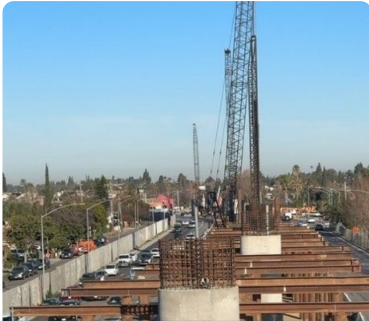
Steel falsework is erected in the median of Capitol Expressway, north of Story Road. (Photo by Mohammad Alazzah).
