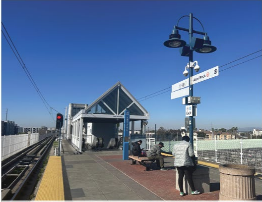
The shade structure is inadequate in providing rain protection
