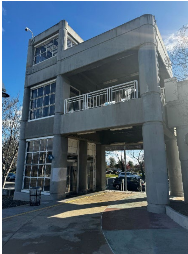
Vertical access to the Great Mall Transit Station from north of Great Mall Parkway is unidentified and lacks clear wayfinding.
