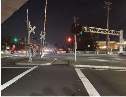
Crosswalk leading to station entry in the median
