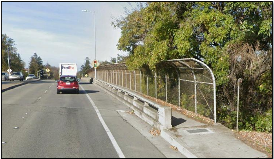
Existing Wolfe Road Overcrossing
