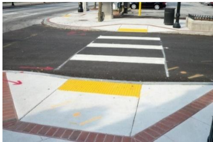
Directional curb ramps
