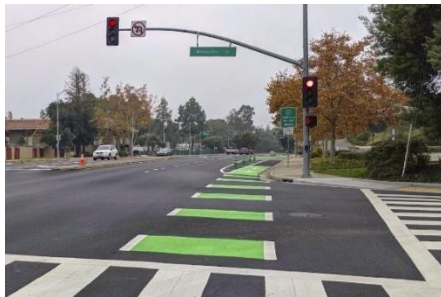
Bicycle lane markings through intersection
