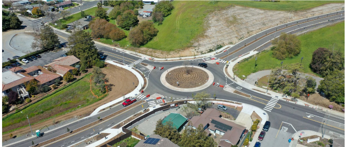
Flyover image of the Santa Teresa-Hale Corridor Rd. Project in the City of Morgan Hill
