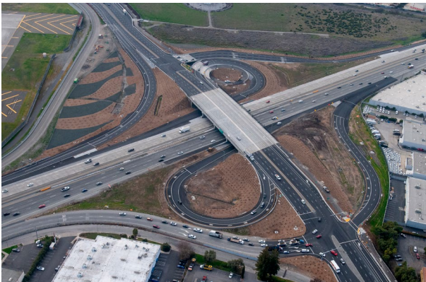
Flyover image of the completed US 101/De La Cruz Blvd./Trimble Rd. Interchange Project in the City of San Jose
