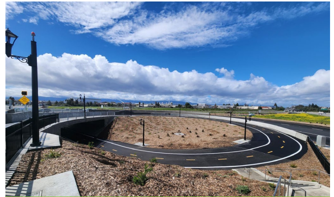
Multi-use path for bicyclists and pedestrians as part of the US 101/De La Cruz Blvd./Trimble Rd. Interchange Project in the City of San Jose
