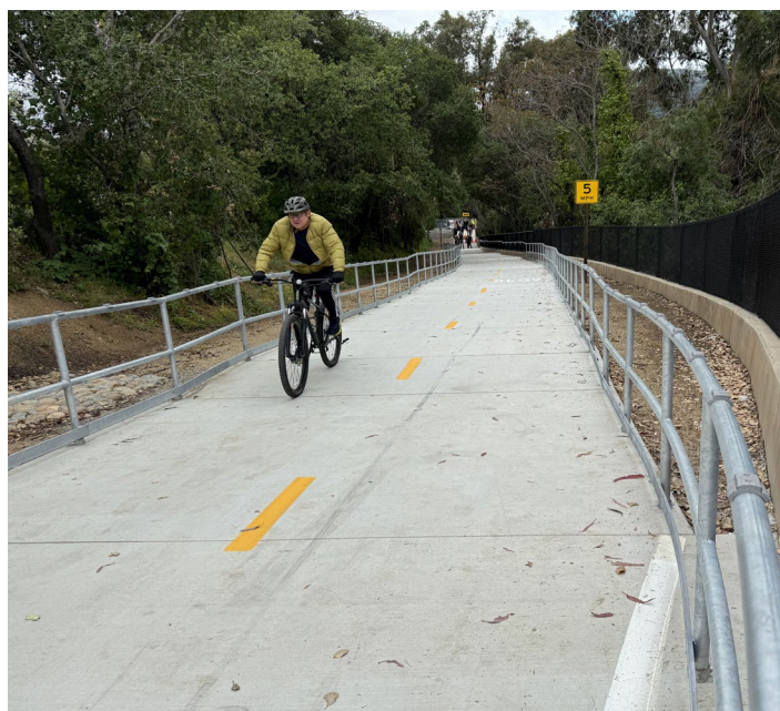
A new pathway for pedestrians, bicyclists, and other trail users as part of the Los Gatos Creek Trail Connector to Highway 9 Project in Los Gatos
