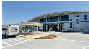
BART Station Entry BART Station車站入口 / Lối Vào Ga BART
