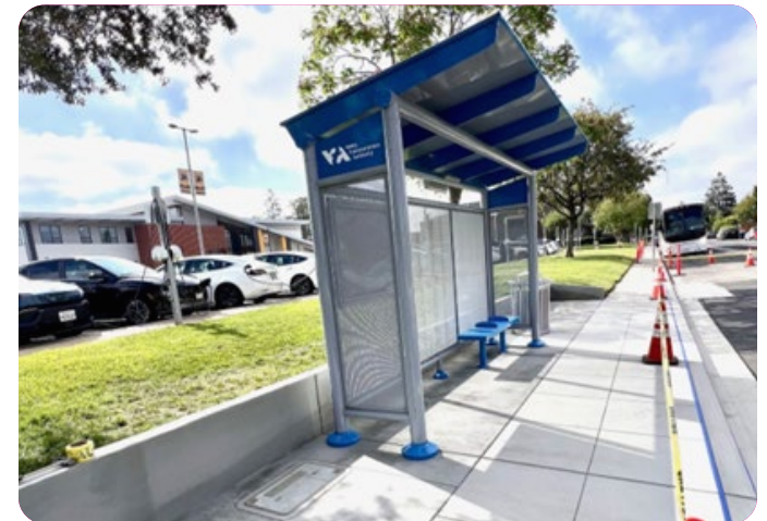
Bus stop at N. Truman Avenue and Bryant Avenue (After)
