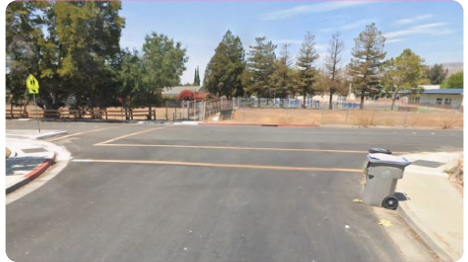
School crosswalk enhancement on D'amico Ave in the City of San Jose (Before)
