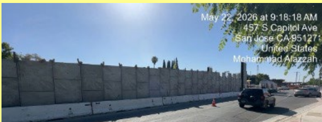
MSE wall at the north end of the project, on northbound Capitol Avenue, approaching Westboro Drive.
