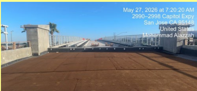
The abutment at the south side of the project. The bridge extends north, and the ramp will land at the future Eastridge Station.
