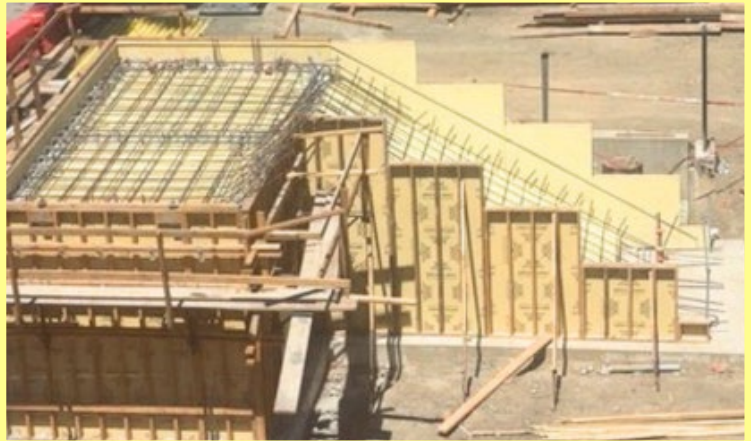
The lower portion of the stairs structure, east side of the future VTA Story Road Station.
