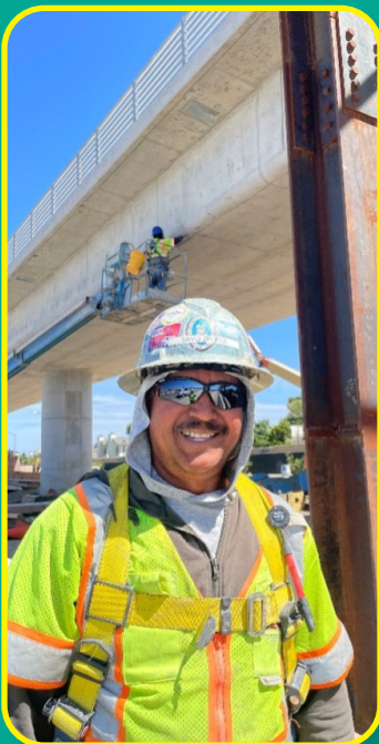
David Zecena, a foreman with the Masons Union, with his crew grinding and patching the finished structure, south of Ocala Avenue.
