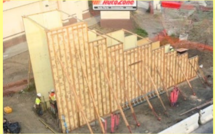
These foundations located on the west side of the project will support access to the future VTA Story Road Station.
