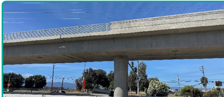
A section of the superstructure features, to the left, an ornamental fence where the adjacent areas are not inhabited; and to the right, a sound barrier to mitigate noise to residents living nearby. (Photo by Lupita Franco Peimbert).
