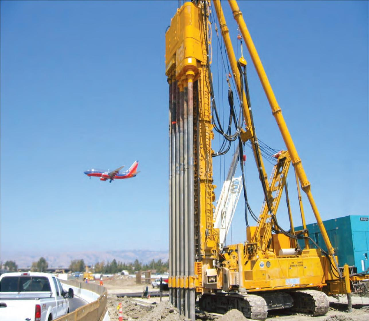
Figure 6-16: Deep Soil Mix and Auger Rig Installation
