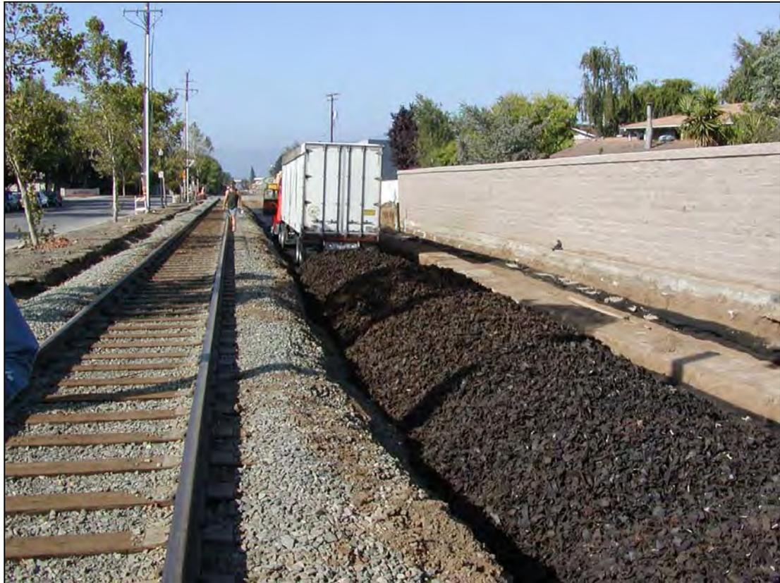
**Figure 3.12-6. Application of Tire-Derived Aggregate Along the Vasona Light Rail Line**
