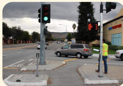
Adaptive pedestrian signals allow for the extension of the pedestrian crossing interval to accommodate slower walking pedestrians.
