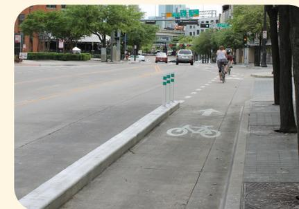
Vertical separation elements, such as flexible bollards, enhance the visual separation between the vehicle travelway and bicycle lane.
