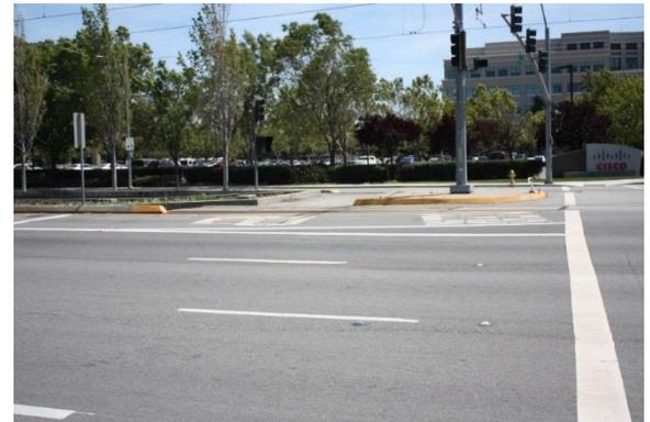
Photo 21: The pedestrian refuge from the Cisco Way Station does not connect to the marked crosswalk
