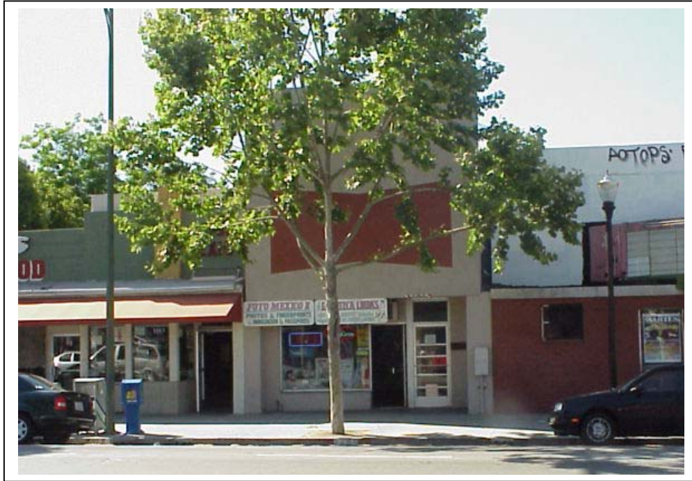
Photograph 2. Camera facing north, May 30, 2002.
