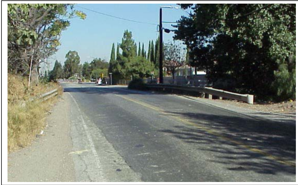
Photograph 2. Bridge deck, camera facing north, September 18, 2002.
