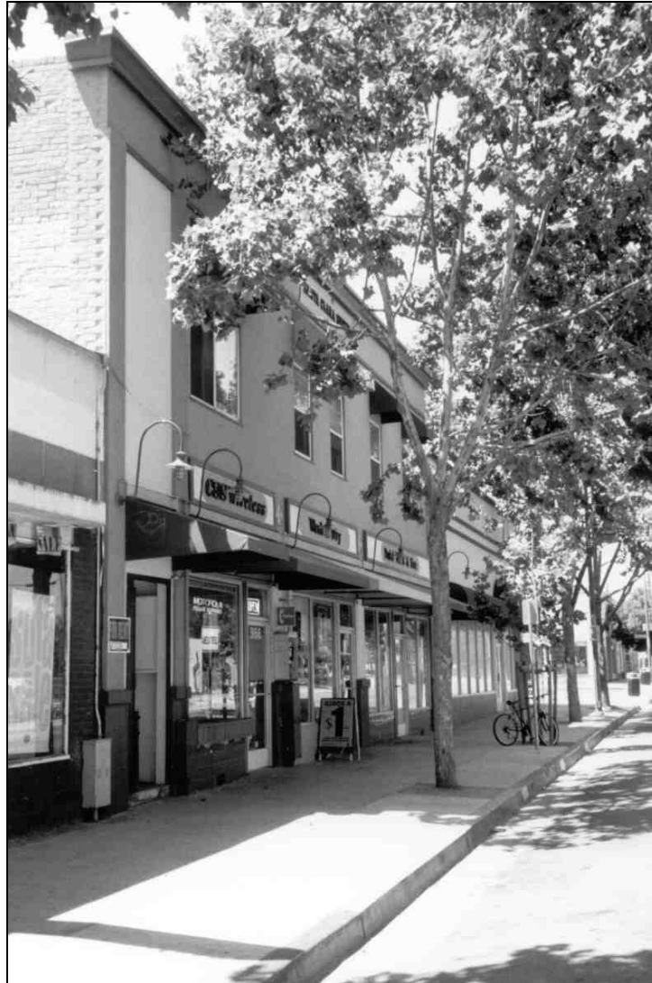
E. Santa Clara Street façade
