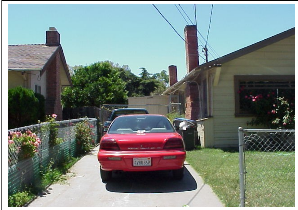
Photograph 2. Addition on the south side, camera facing west, July 24, 2002.
