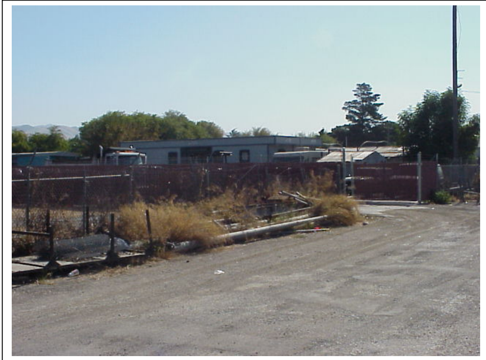
Photograph 2. Small sheds and modern manufactured buildings, camera facing southeast, October 3, 2002.
