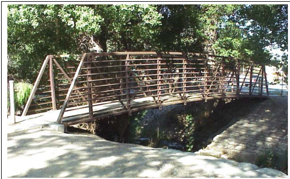
Photograph 3. Footbridge east of Upper Penitencia Creek Bridge, camera facing northwest, September 18, 2002.
