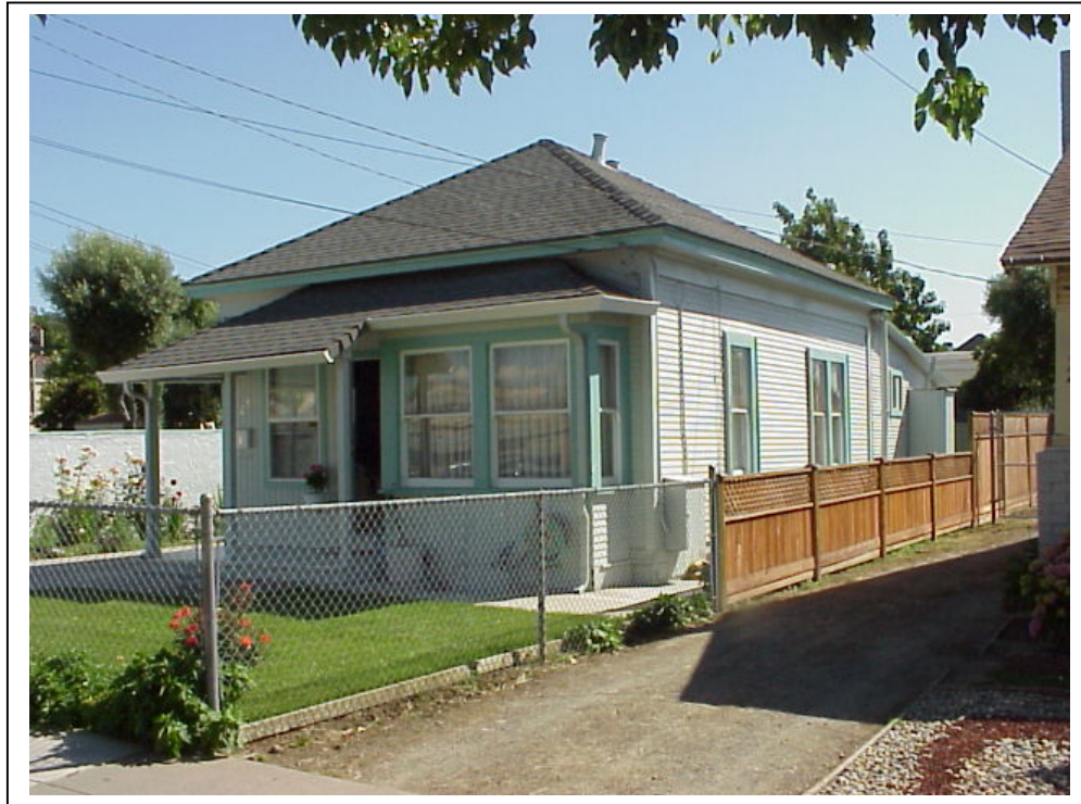
Photograph 2. East and north sides, camera facing southwest, May 30, 2002.
