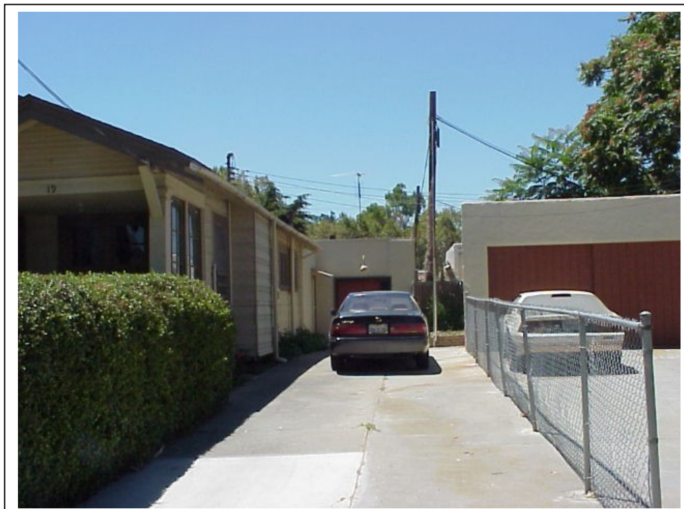
Photograph 3. Addition on the north side, camera facing west, July 24, 2002.
