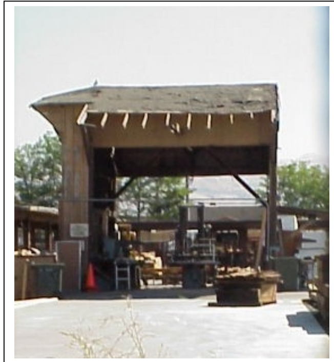
Photograph 3. Building D, camera facing east, July 23, 2002.
