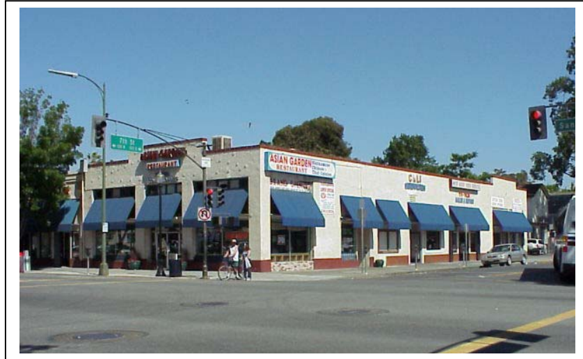
Photograph 1. Façade, camera facing east, May 2002.
