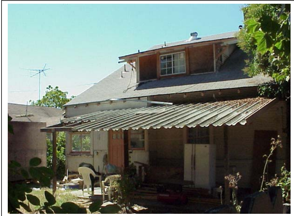
Photograph 2. East side of house, camera facing southwest, September 17, 2002.
