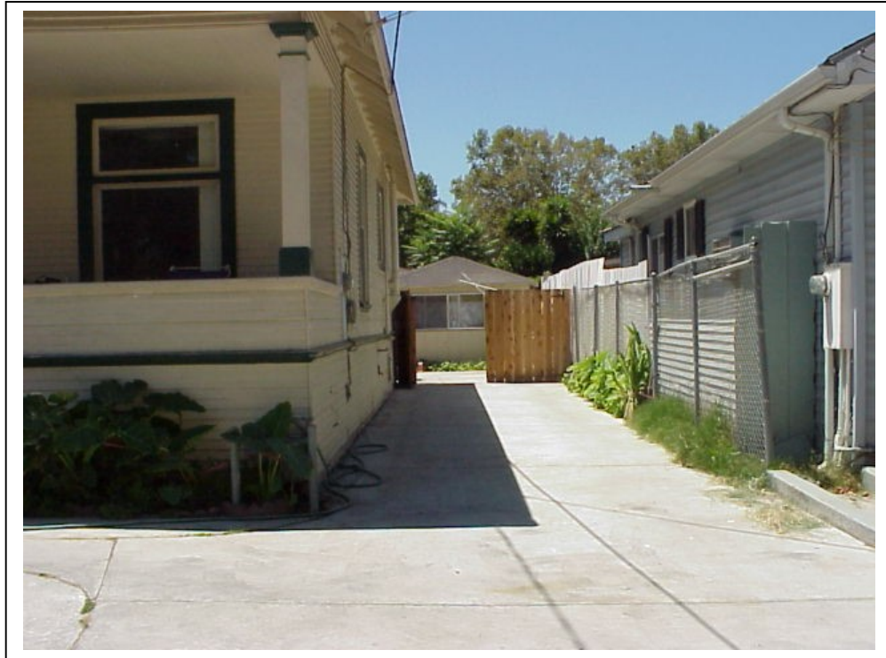
Photograph 2. View of east side of converted 1951 detached garage, July 23, 2002.
