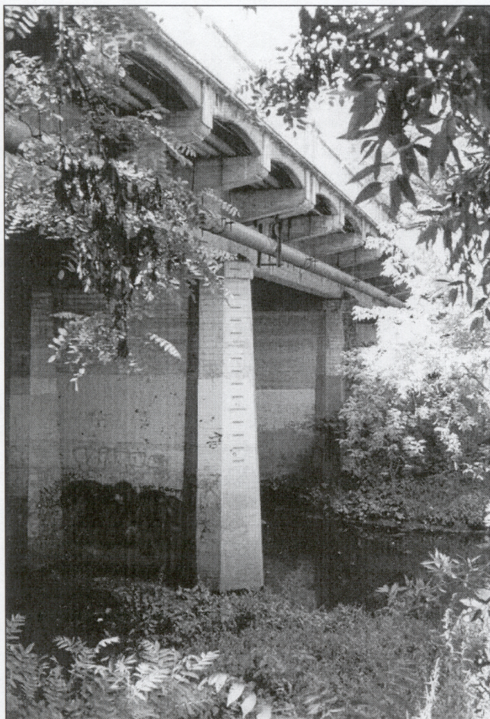
View of superstructure
