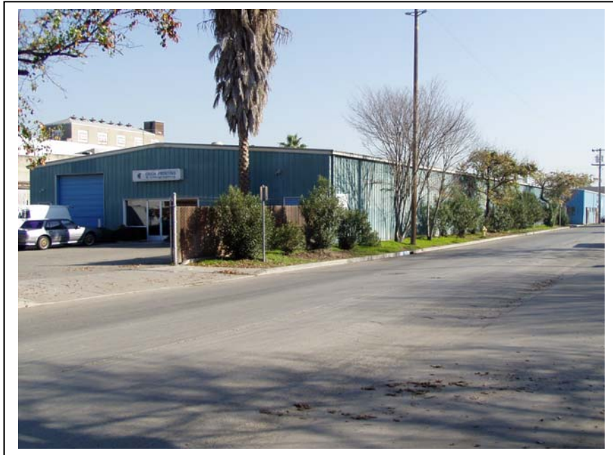
Photograph 2. Two modern buildings at north end of parcel, camera facing southeast, January 7, 2003.
