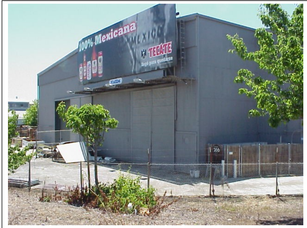
Photograph 2. East side of the building, camera facing west, May 30, 2002.
