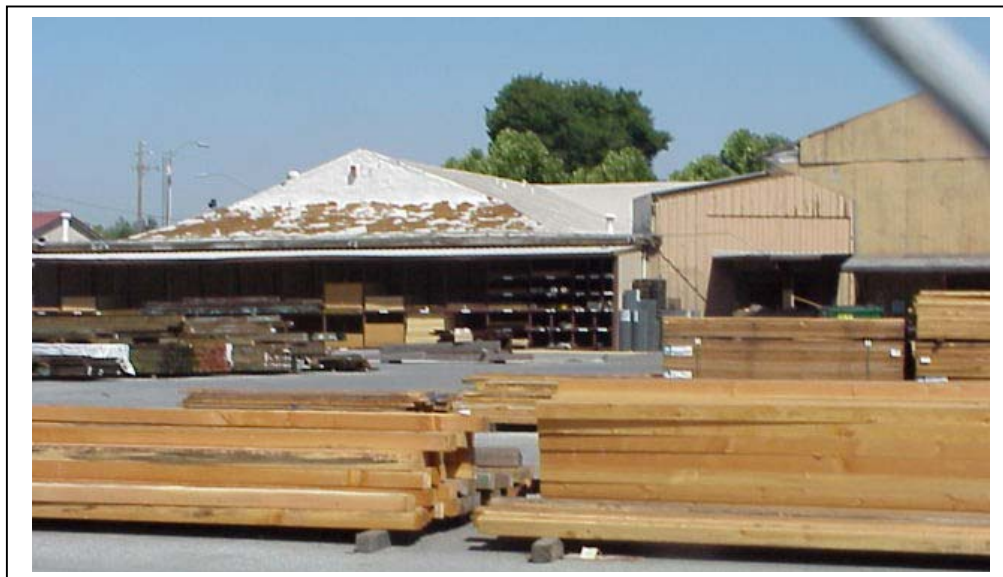
Photograph 2. Buildings A (left), B (right rear), and D (right foreground). Camera facing north, July 23, 2002.
