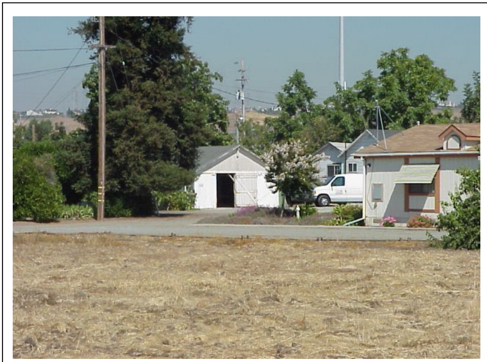
Photograph 3. Garage, camera facing northeast, September 25, 2002.
