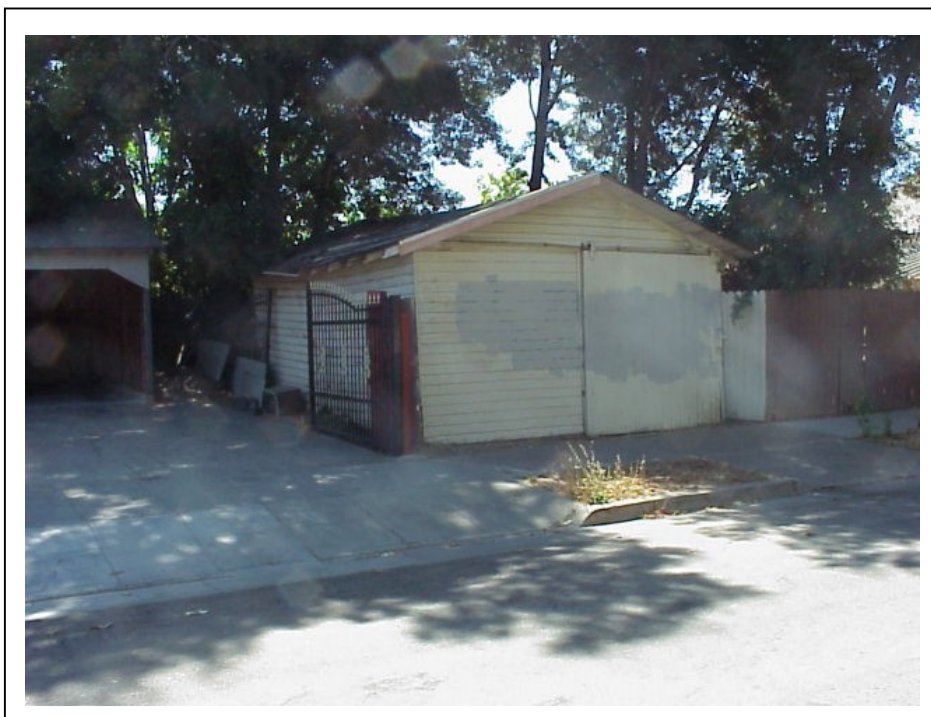
Photograph 3. Detached garage, camera facing southwest, September 17, 2002.
