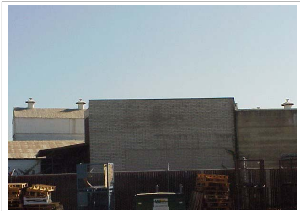
Photograph 3. Area B, camera facing east, September 20, 2002.
