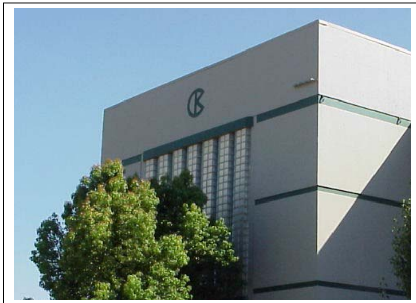
Photograph 2. Front detail, camera facing northeast, July 23, 2002.
