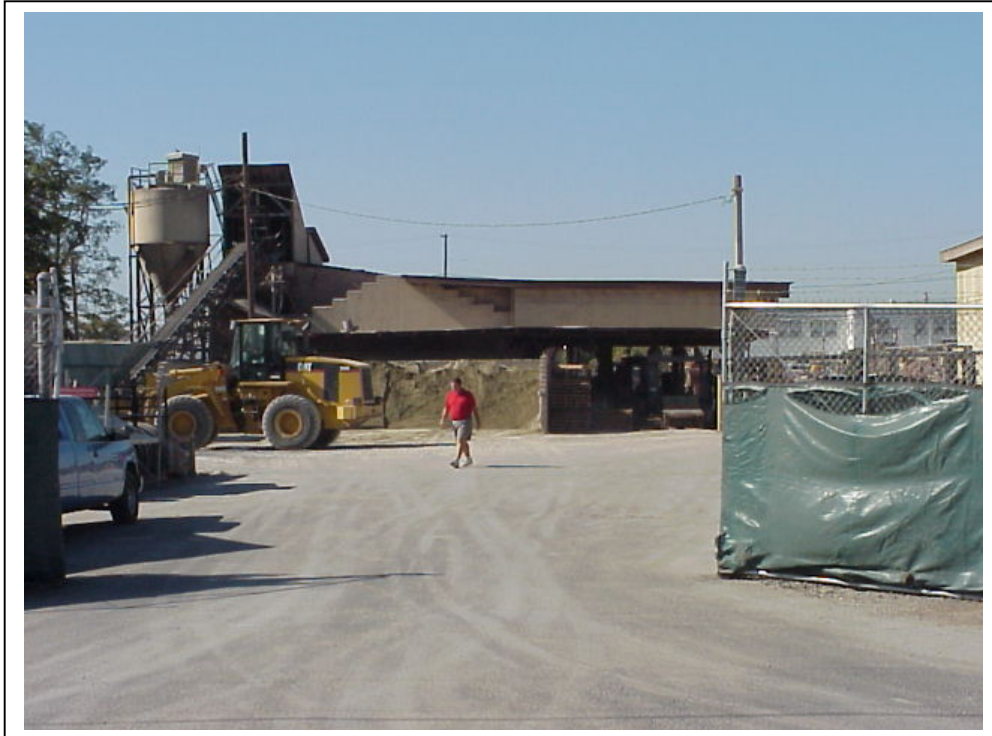
Photograph 2. Historic concrete works, camera facing southeast, October 3, 2002.
