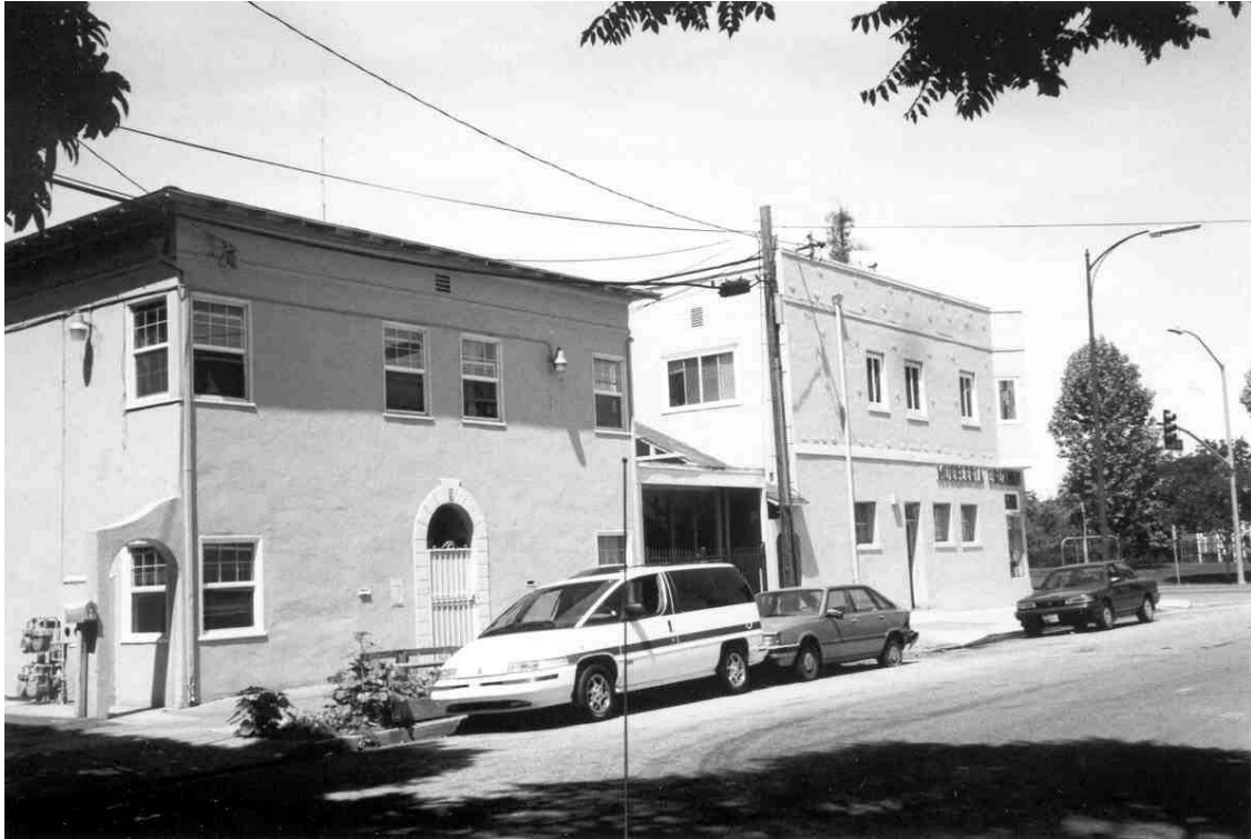
South 19 th Street façade
