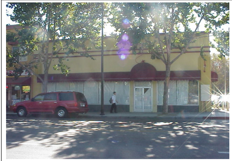
Photograph 1. Façade, camera facing southeast, October 3, 2002.
