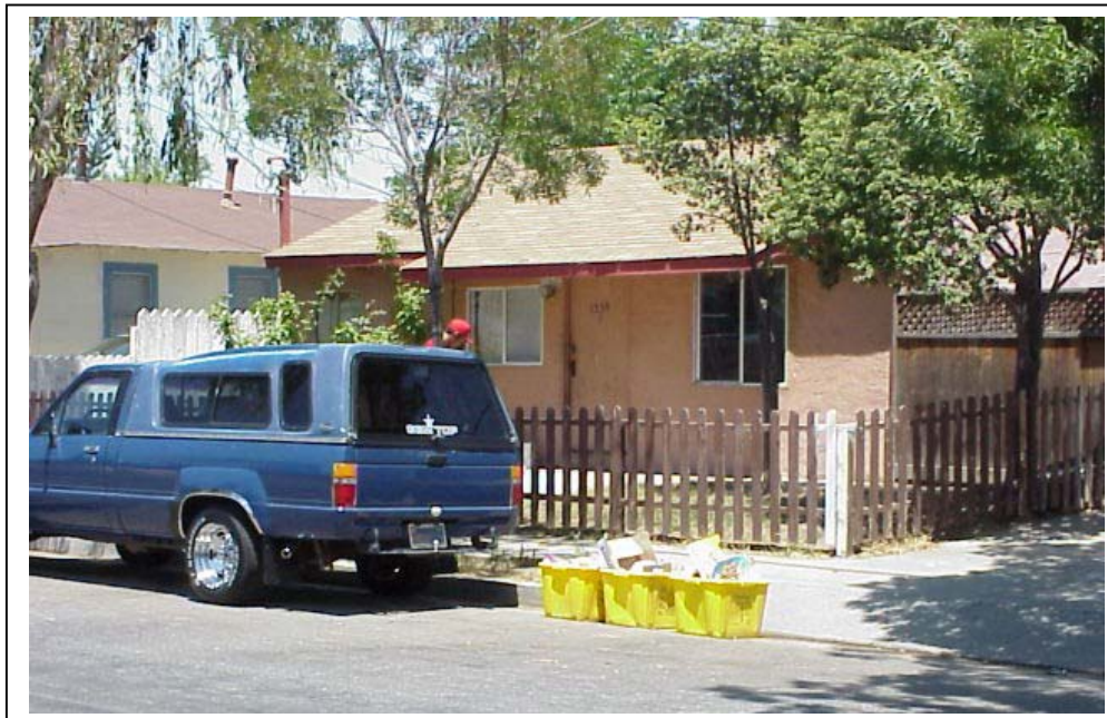
Photograph 3. Secondary residence, camera facing northeast, July 23, 2002.
