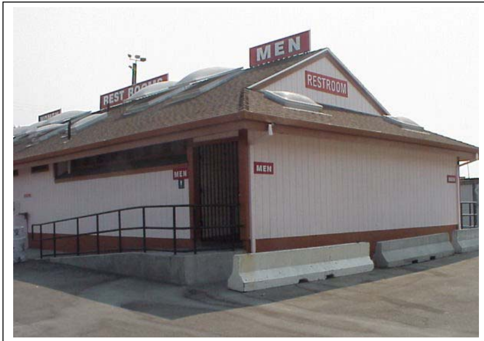
Photograph 4. Restroom, camera facing southeast, August 15, 2002.
