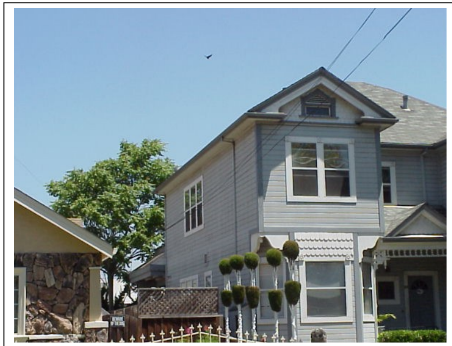
Photograph 2. View of additions, camera facing southeast, July 23, 2002.
