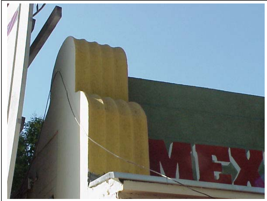
Photograph 2. Camera facing north, May 30, 2002.
