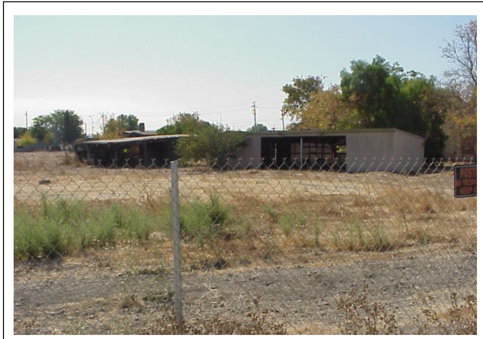
Photograph 4. Wood frame sheds, camera facing southwest, September 25, 2002.
