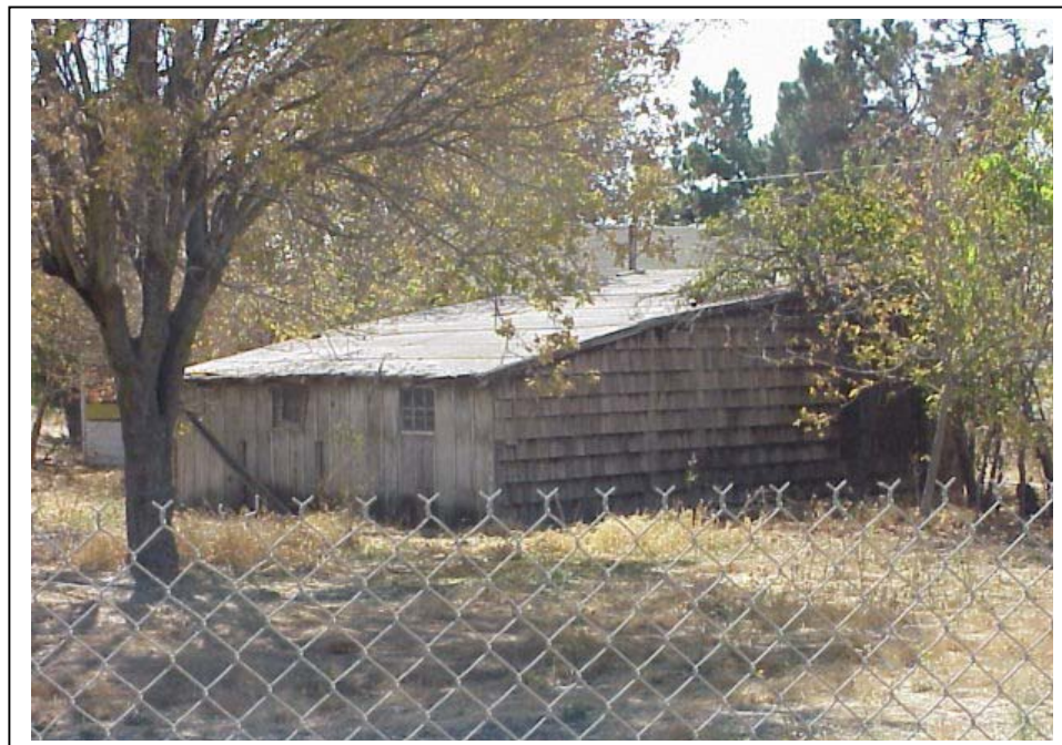
Photograph 3. Garage, camera facing southwest, September 25, 2002.
