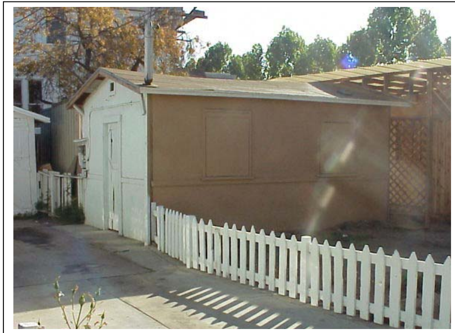
Photograph 2. Original commercial building, camera facing east, September 17, 2002.
