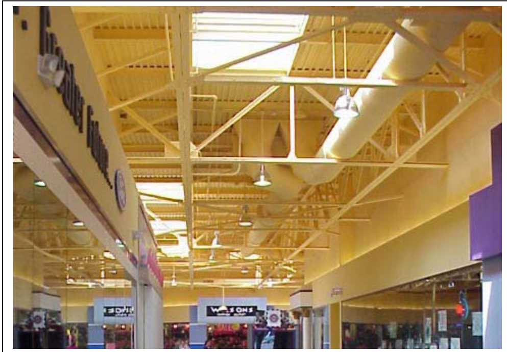
Photograph 6. Interior of Great Mall, reflecting remnants of roof truss of Ford Motor Assembly Plant, July 2002.
