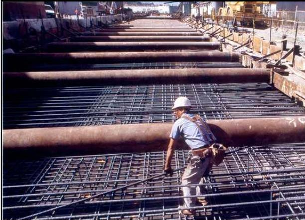
**Figure 4.19-15: Installation of Station Roof**
