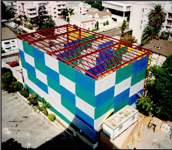
**Figure 4.19-28: Construction Site Screening Example #1**
