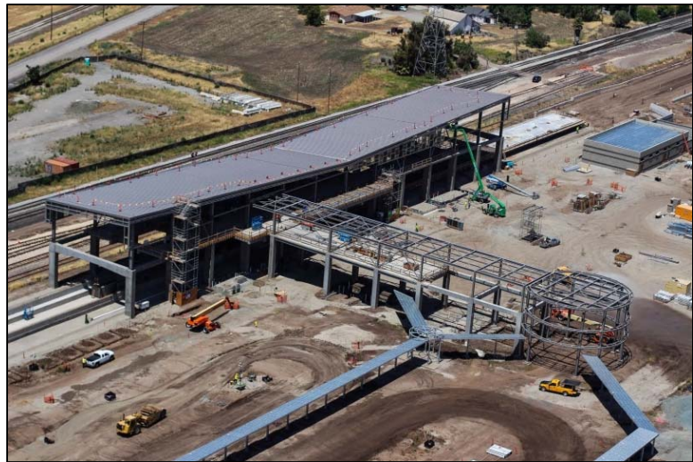
Warm Springs / South Fremont Station Construction
