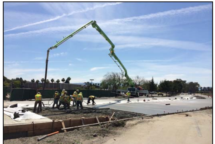
Concrete pour on the north section of the new loop road
