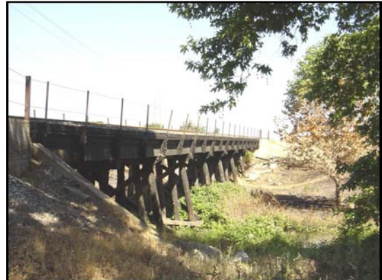
Llagas Creek Bridge
