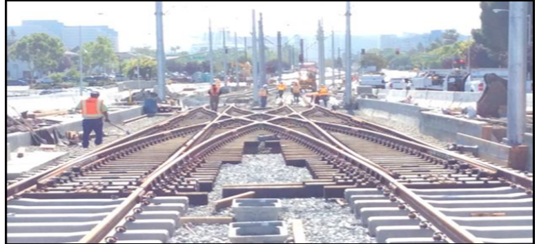
Double Crossover installation for the new Santa Clara Pocket Track
