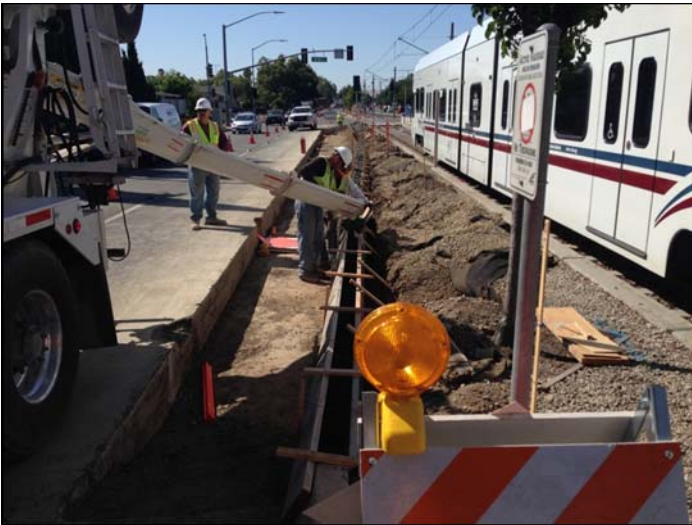
Roadway reconfiguration on Capitol Ave. near Alum Rock Station
