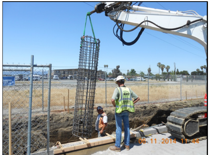
Pile foundation for platform at Ocala Bus Station
