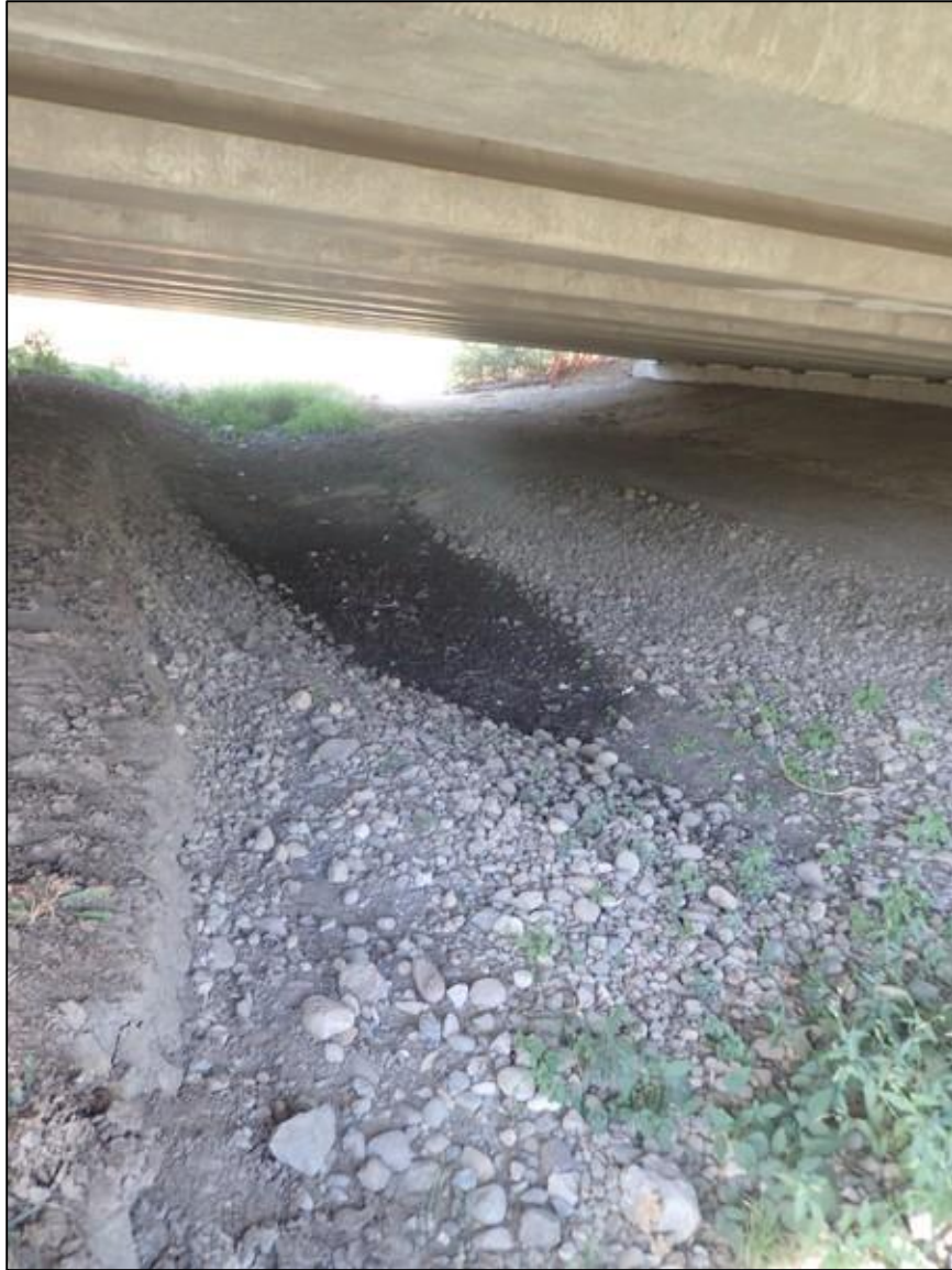
Photo 5. Damp channel in Habitat Unit 4 (fall 2015)
