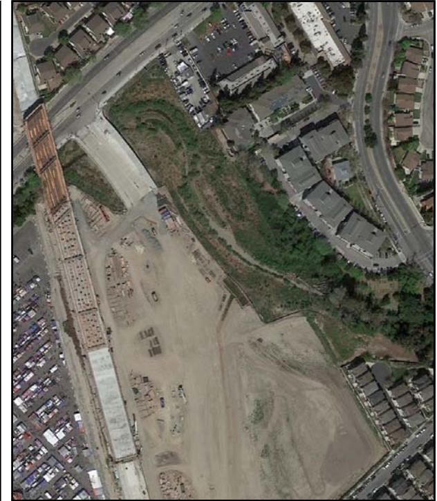
C. March 2015, 3 years after channel construction.
