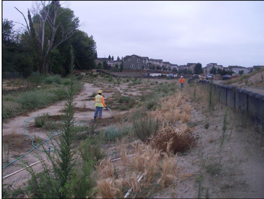
Photo 3. Photodocumentation Point 5A, looking east at the Upper Floodplain Planting Zone along the western boundary of the mitigation site (August 28, 2013)
