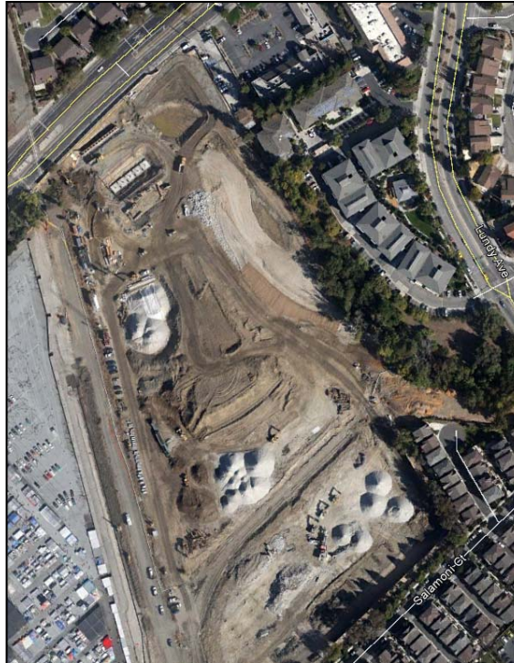
B. September 11, 2012, Channel construction period
