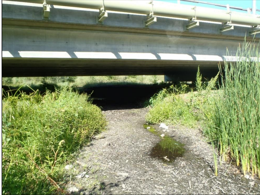
Photo 3. Damp channel and standing water in Habitat Unit 4, looking upstream (fall 2015)
