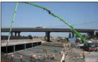
*Concrete placement for the invert slab of Berryessa Creek box culvert*
