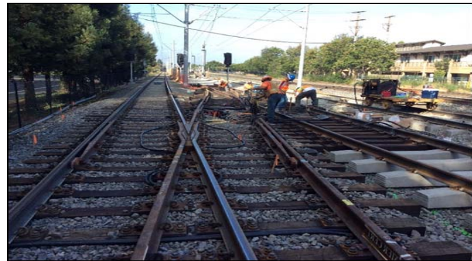
Turnout and switch machine installation in progress near Stevens Creek Bridge
