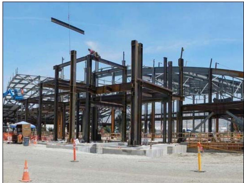
Installation of Steel for the Pedestrian Overcrossing at the Milpitas BART Station
