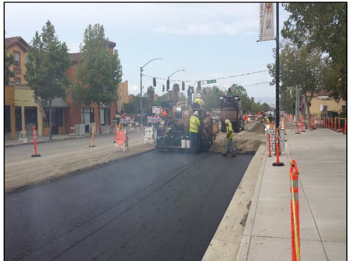
Roadway work in progress on Alum Rock Avenue
