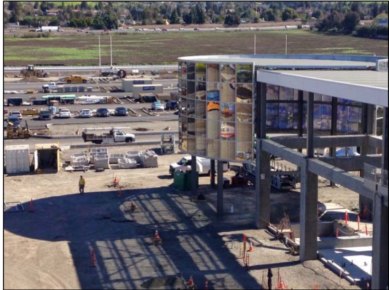
Warm Springs / South Fremont Station Entry Pavilion art glass installation
