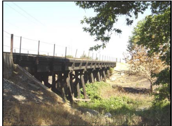
Llagas Creek Bridge
