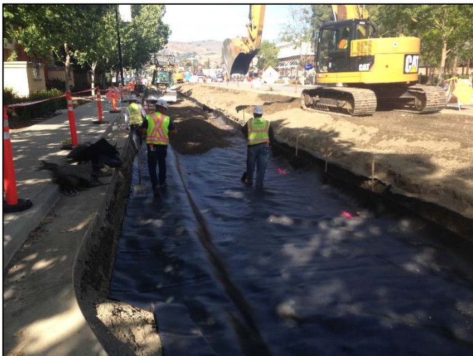
Roadway construction operations on Alum Rock Avenue
