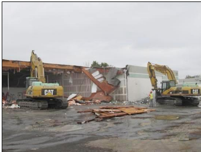
Building Demolition (C700)
