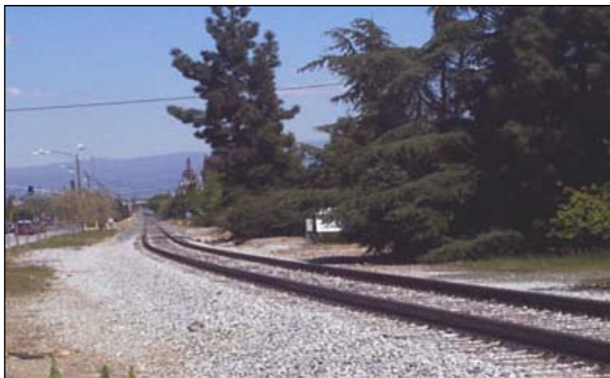
View of Proposed Alignment Looking North from the Route 85 Terminus
