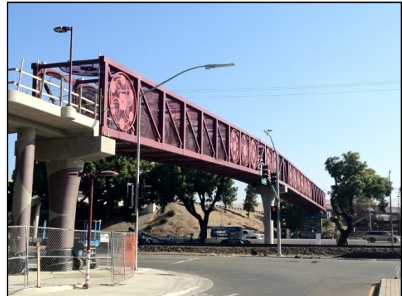
Blossom Hill Pedestrian Bridge Installed
