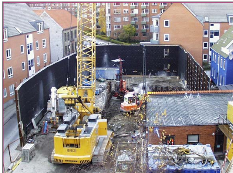
Figure 4.19-29: Construction Site Screening Example #2
