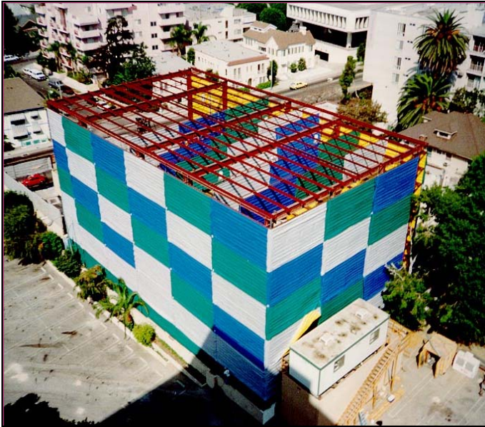
Figure 4.19-28: Construction Site Screening Example #1
