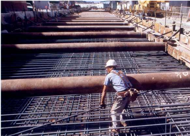
Figure 4.19-15: Installation of Station Roof
