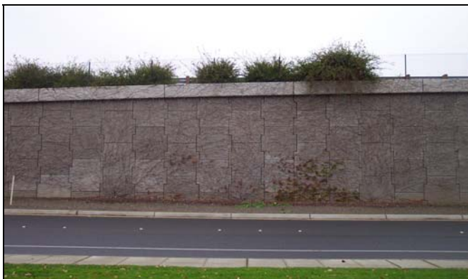
Figure 4.19-3: Example of Mechanically Stabilized Wall
