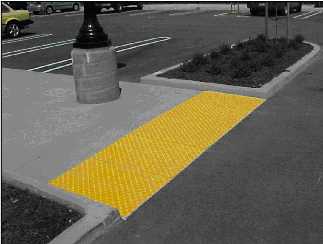
**Figure 38: Detectable Warning Band at edge of pedestrian path adjacent to vehicular roadway
