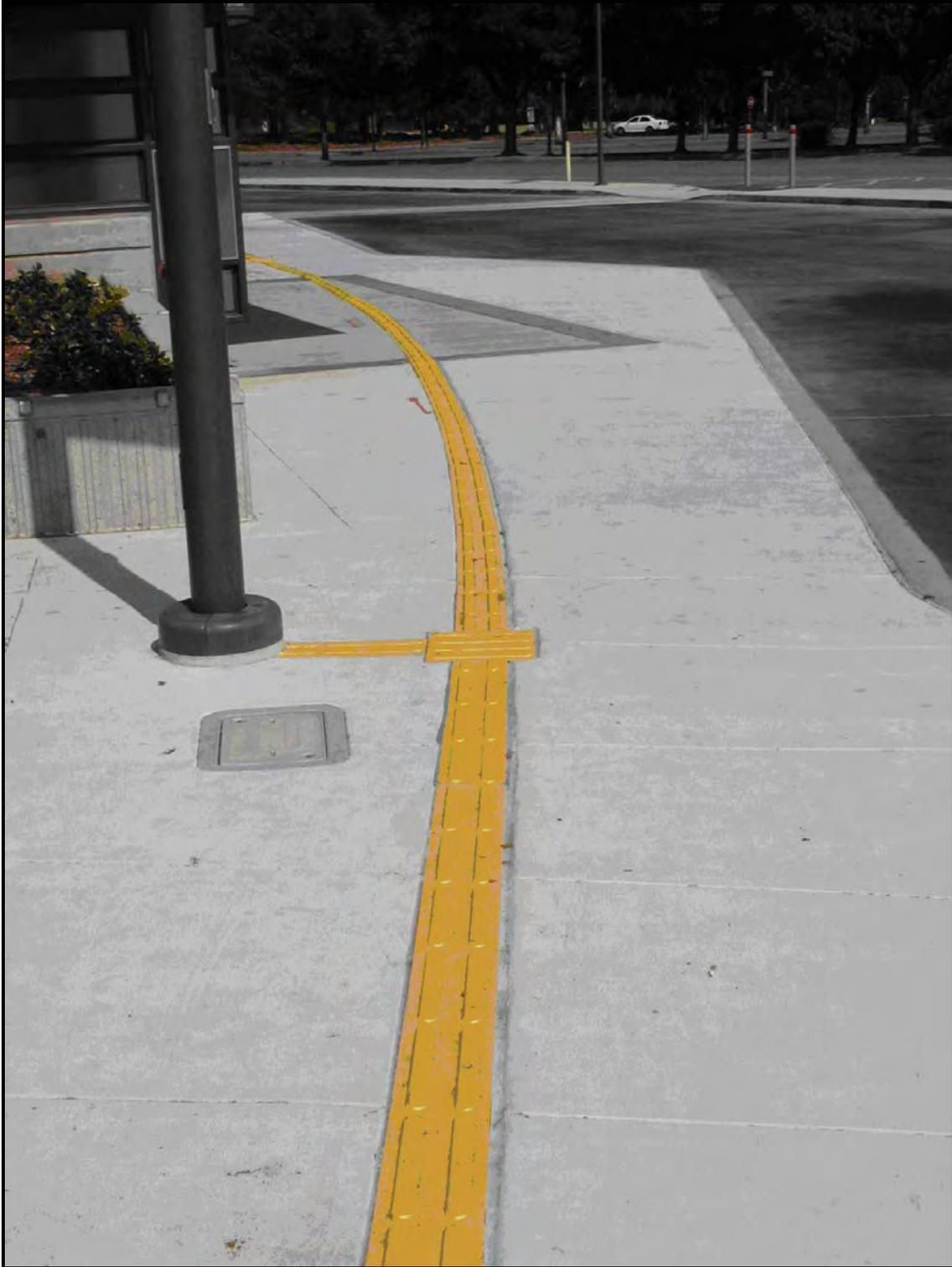
**Figure 31: Directional Bar Tile with Decision Tile leading to an electrolier used as a bus stop pole.
