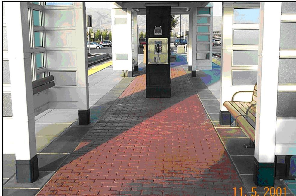
**Figure 37: Example of mixed use of walking surfaces and aesthetic paving in center of light rail platform with larger pavers in the designated accessible path along the platform edge. Location: I-880/Milpitas Light Rail Station.**
